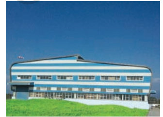
Specialty Bldg.; Himachal Pradesh 1,20,000 sqft
